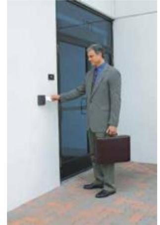
*A user is trying to open the door by placing an RFID tag near the RFID reader*
